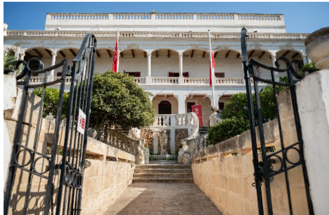
Villa Portelli, Kalkara, Malta - one of the HERITALISE Project Use Cases
